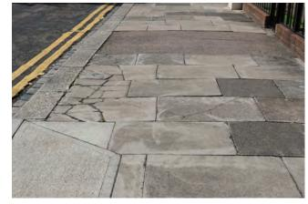
Cracked paving slabs
