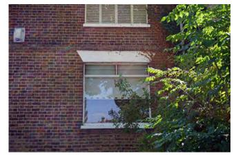
Window frame of timber but with inappropriately proportioned glazing bars
