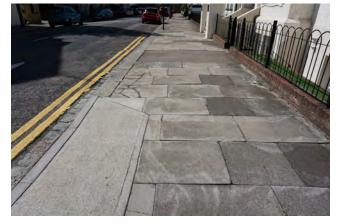
Cracked concrete slab paving. Note granite kerb stones and cobbled gutter
