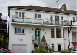
Glazed balconies, infilled recessed porch and sunken driveway for a garage are inappropriate alterations to this house
