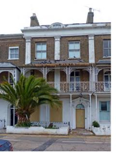
Vacant building on the Royal Terrace, suffering from poor condition, such as blocked gutters and deteriorating timberwork
